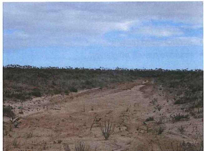
Figure 1. A poorly maintained roaded catchment with weed growth evident, and erosion leading to deposition of silt at the collecting end.
