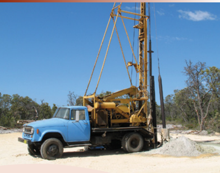
Water drilling rig.
