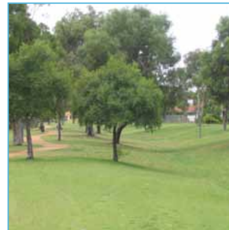
Grassed swale, Allinton Park, Ballajura
