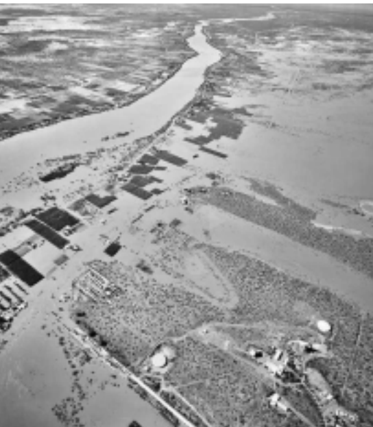
CARNARVON - Looking upstream from Brown Range during 1980 Gascoyne River flooding.
