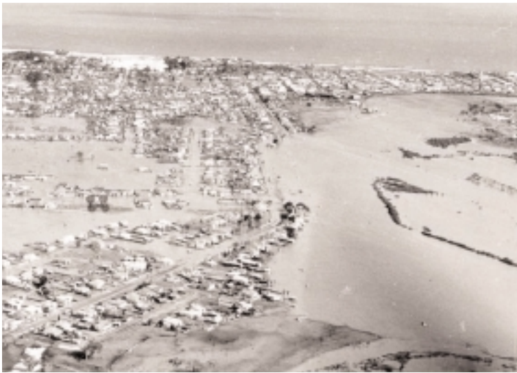
BUNBURY - Preston River levees breached during 1964 flooding.
