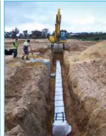
Infiltration trench backfilling, Meadow Springs, City of Mandurah
