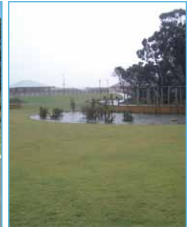
Infiltration basin, flush kerb swales, retained trees, Seasapes, City of Mandurah, after a storm
