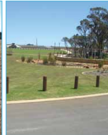
Infiltration basin, flush kerb swales, retained trees, Seasapes, City of Mandurah, before a storm
