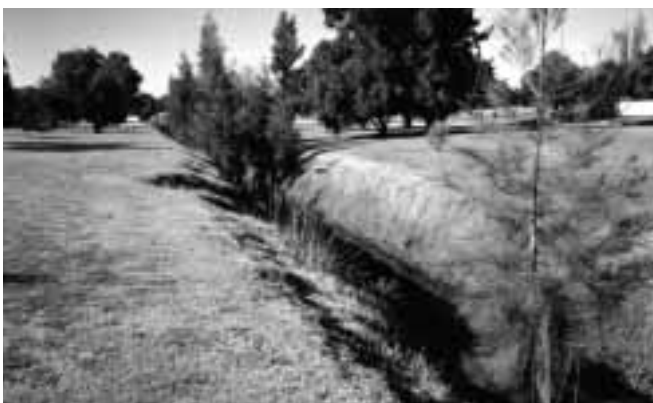
Figure 14. Bannister Creek prior to restoration works.
